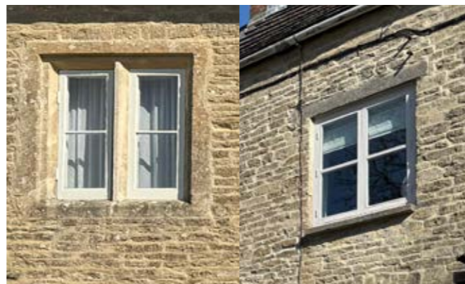
Fairly small well-spaced windows with stone mullion surrounds or set below a stone or timber lintel
