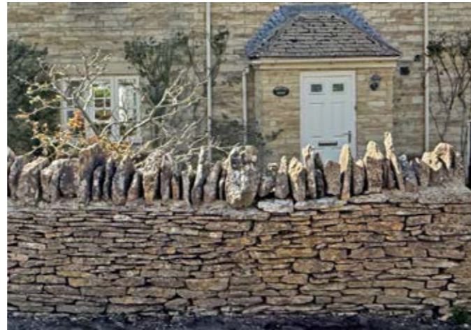
Dry stone walls with cock and hen capping
